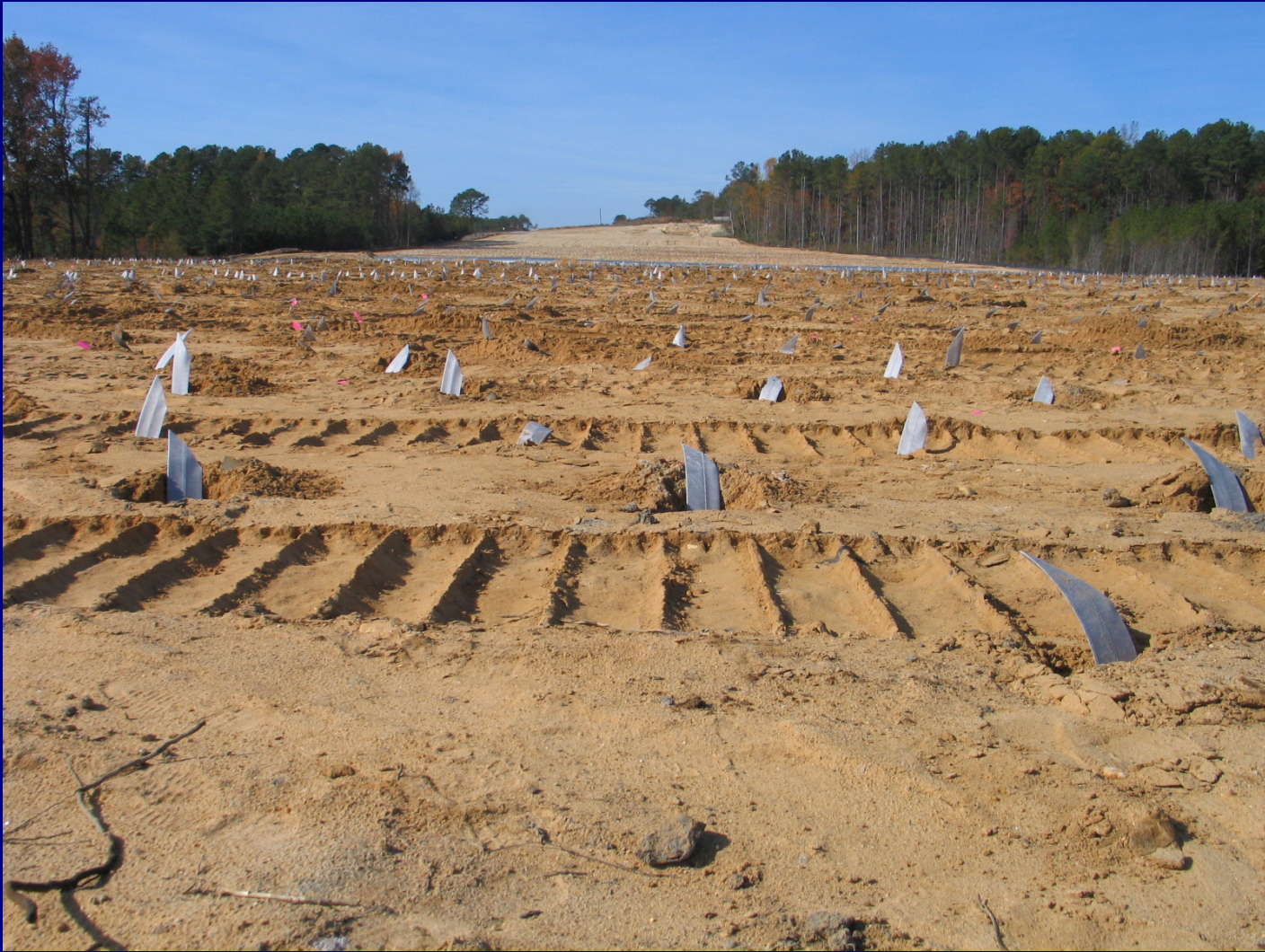
Wick Drain Installation
